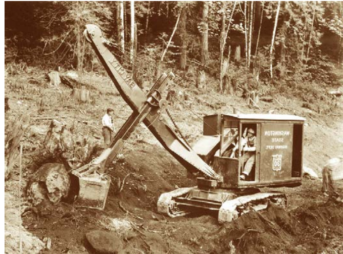
Road Construction circa 1930s - WSDOT
