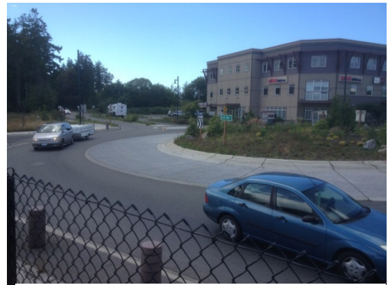
Sims Way (SR 20) Roundabout
