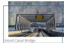
Hood Canal Bridge
