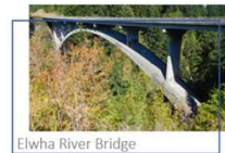
Elwha River Bridge
