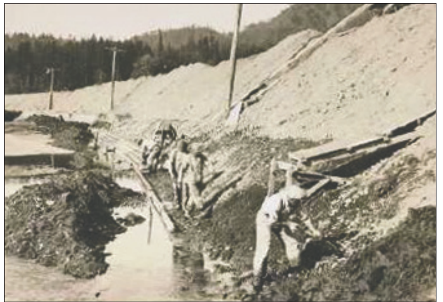
This photo from the 1930s shows the riprap wall that underlies US Highway 101 through the Duckabush Estuary under construction. Photo courtesy of the Washington State Department of Transportation
