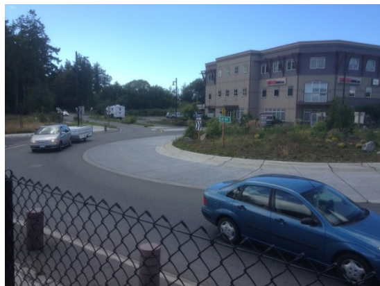
Sims Way (SR 20) Roundabout
