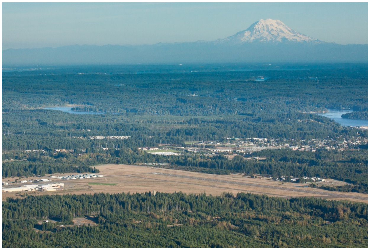
Sanderson Field, Mason Co (with Mt Rainier in background)
