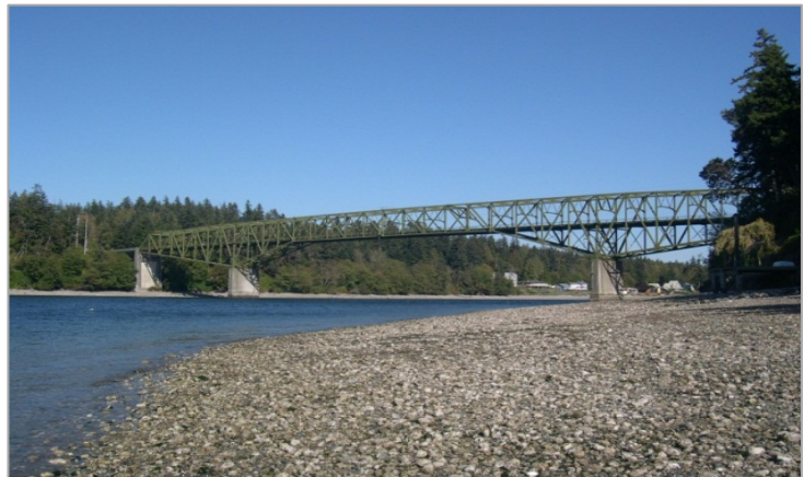
Agate Pass Bridge; Source WSDOT
