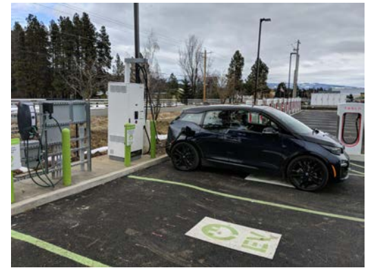
Cle Elum (I-90) Coffee Company (co-located w/ Tesla Supercharger, includes 4.5kW solar array)
