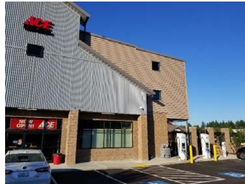
DuPont Ace Hardware (2 DCFC, 1 L2 EVSE)
