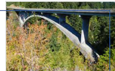
Elwha River Bridge
