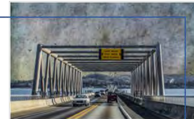
Hood Canal Bridge
