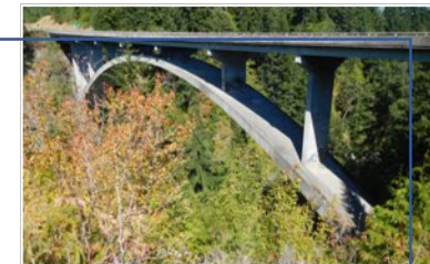
Elwha River Bridge
