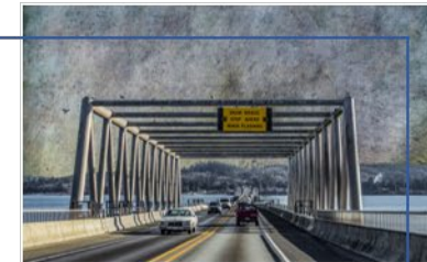
Hood Canal Bridge
