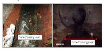
Repair the culvert's failing invert, stabilize adjacent soil and improve fish passage. This is a critical culvert that runs under Lincoln Street and US 101; and it has a high potential for property damage and loss in the event of a collapse. Project cost: \$3.2 million.
